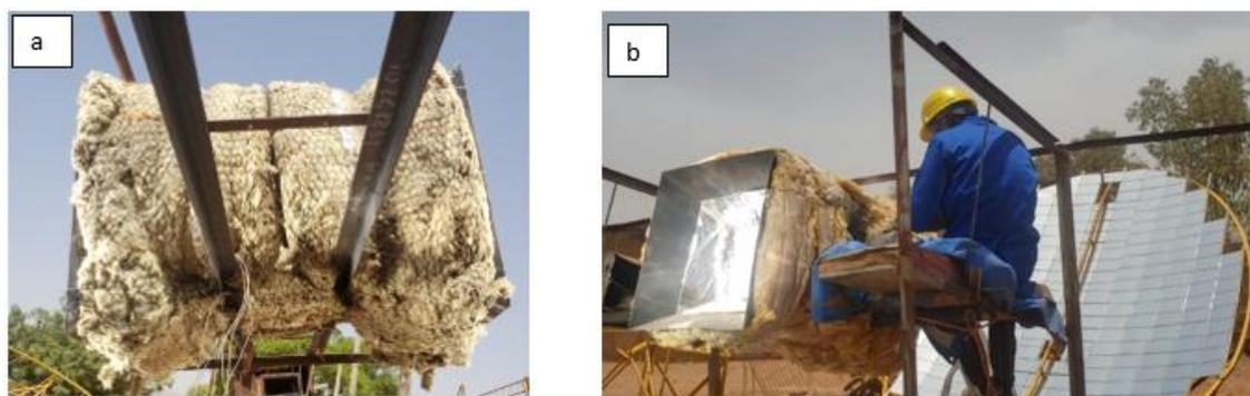
Fig. 3. a) Insulation of the perimeter of the receiver with rock wool. b) Inlet opening of the plastic waste in the receiver
